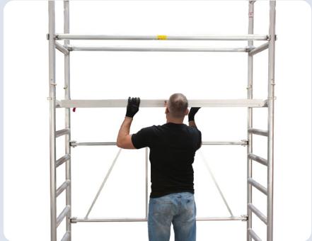
Mount 4 horizontal braces between the railway frames. Now move your platform to the desired height
