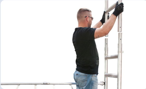
Mount a railway frame at each side and secure with clips
